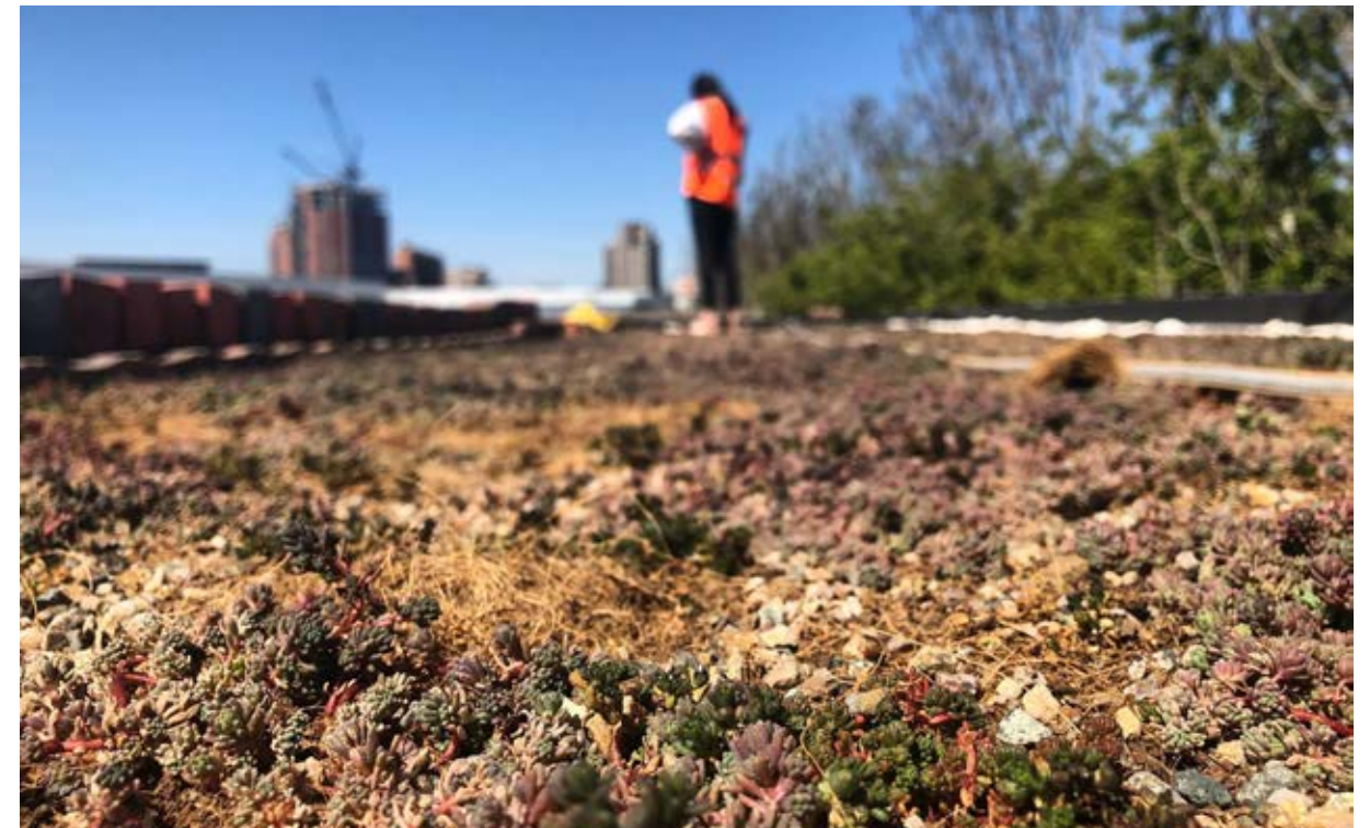
Biodiverse green roof on top of one of our studio containers with exposed substrate.
